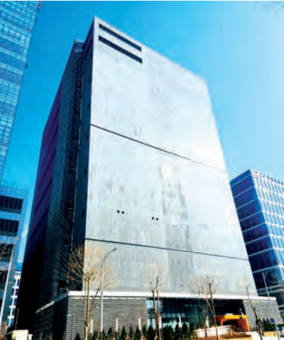
Anyang EPOCH Data Center 40MW (Construction Completed in January 2024)
