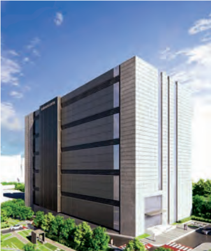
Ilsan Magna Data Center 20MW (Construction Commenced in Nov 2024)
